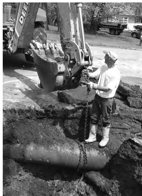
Water and Sewer Department Crews perform an emergency water main repair on West Hanover Avenue.
