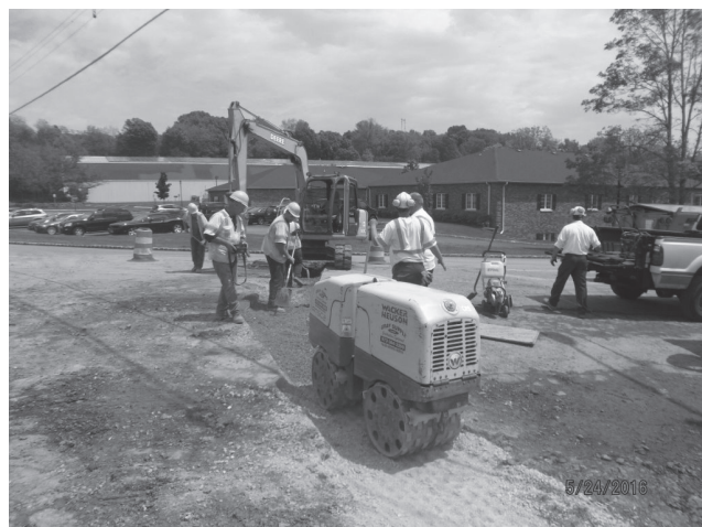
Water & Sewer Department crew works on the realignment of the water main along West Hanover Avenue and Sussex Turnpike.
