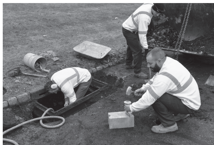
Department of Public Works crew makes repairs to a catch basin.
