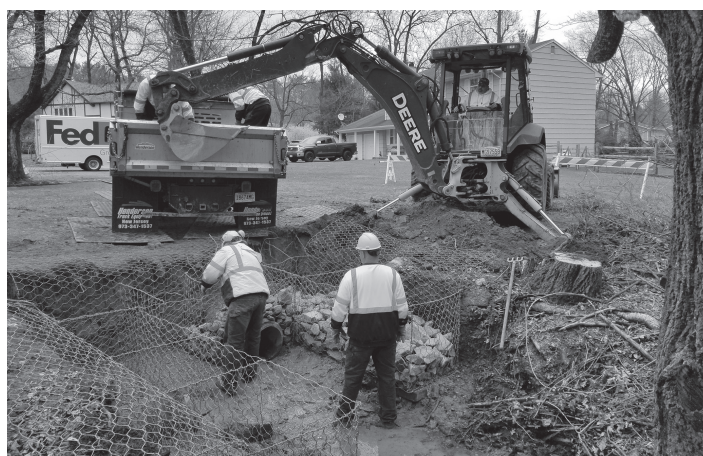
Township Public Works staff install drainage swale for a stormwater management project on Quaker Hill Lane.
